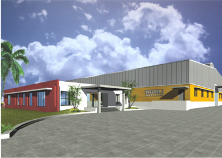
Our New Factory Near Mumbai, India.
